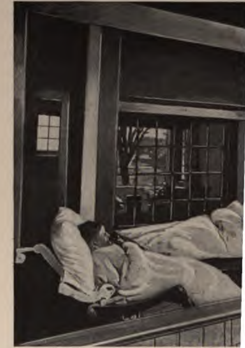
FIG. 328.—Outer wall of house windowed so that bed can be raised to open porch side.
